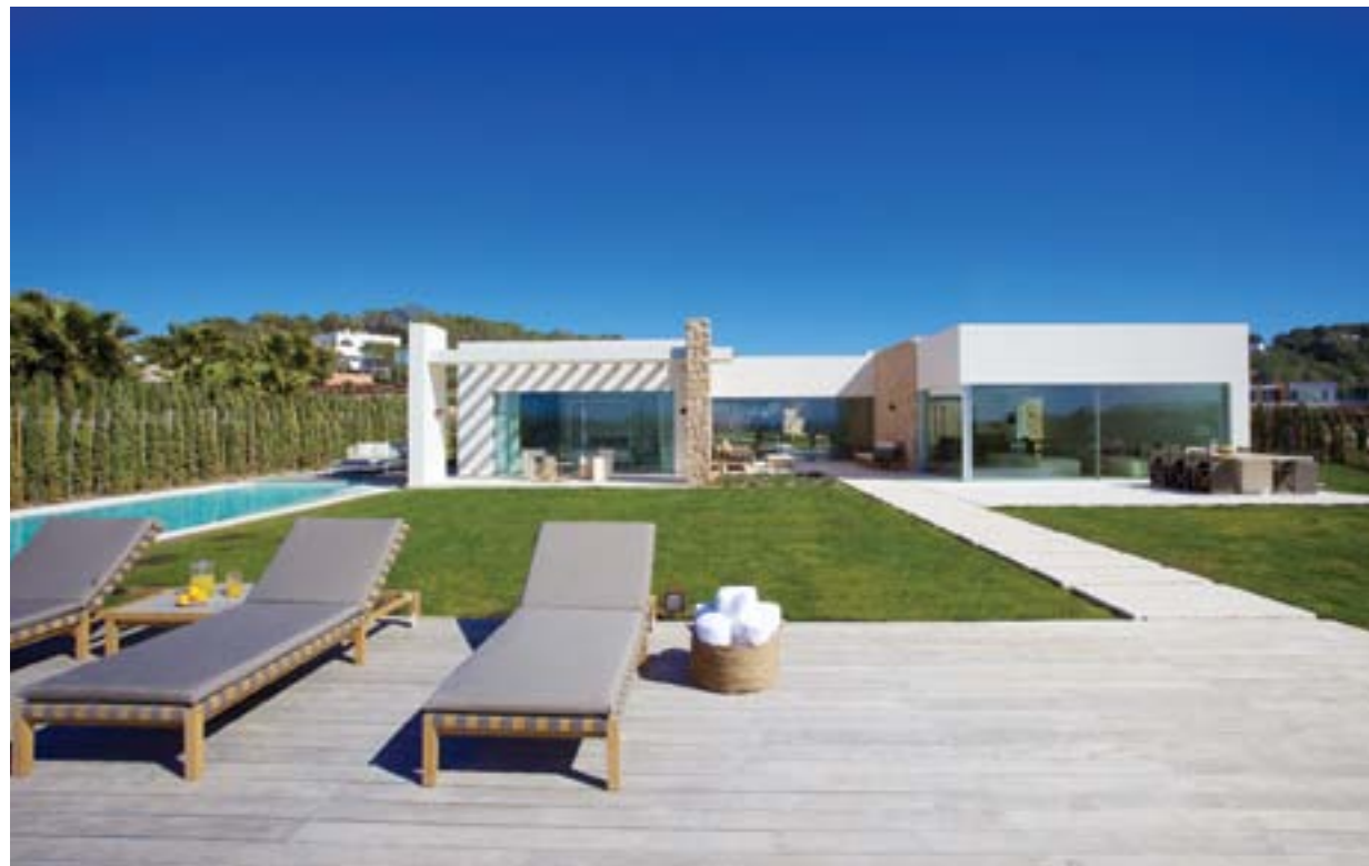
Vista general de Can Dos Rocas / General view of Can Dos Rocas
